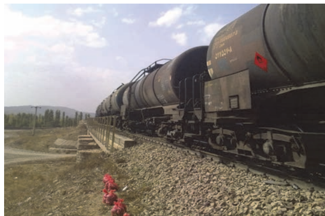
Figure 3. Ballasted railway track
